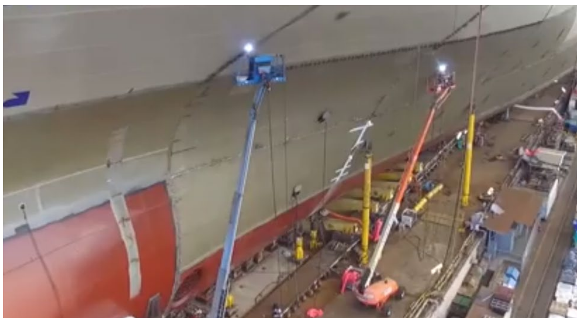
Figure 4-1. Welding on Vessel Hull from Mobile Elevated Work Platforms
