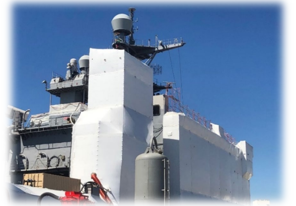
Shrouding for Ship Repair Operations
