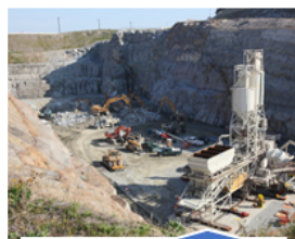
Concrete Batch Plants
